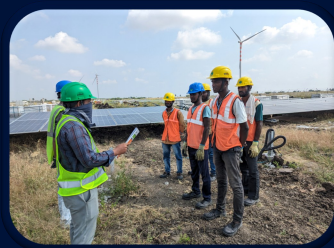
72MW Solar Power plant AMP+ / Essens MMS, Tamilnadu, 2024
